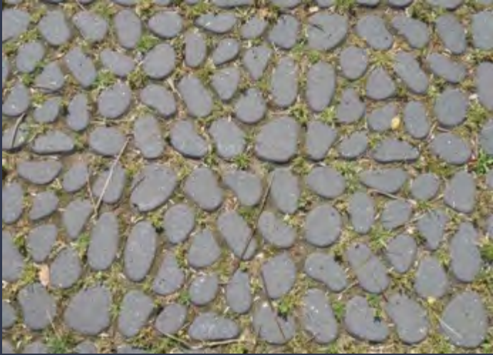
Pavimento permeable (Unalab)
