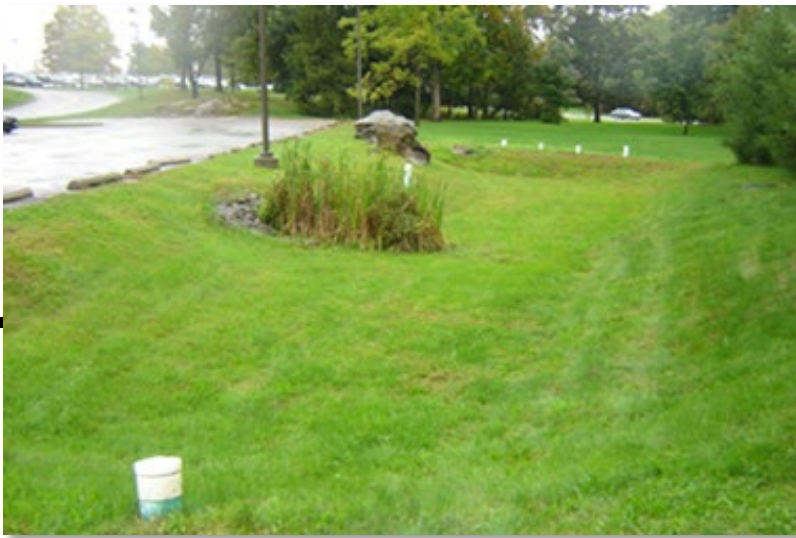
Extended detention basins
